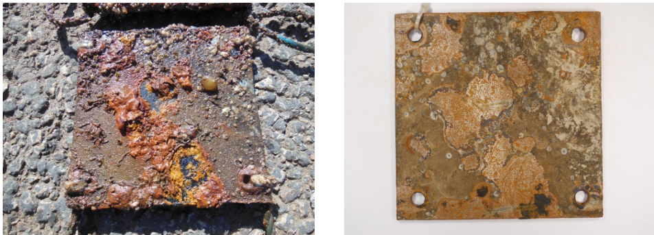
Figure 42 Steel plate before and after cleaning.
