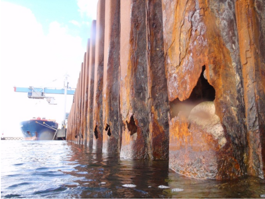
Figure 29 Sheet pile wall on the Swedish west coast suffering from severe corrosion.
