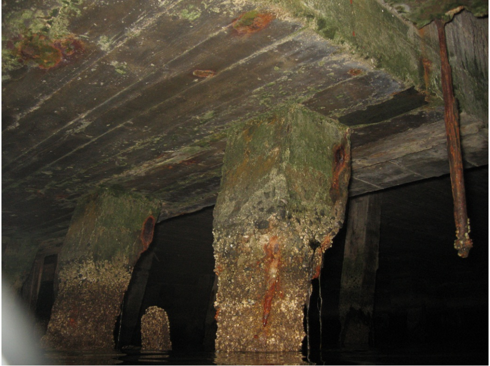
Figure 1 Damages on concrete piles on the underside of a concrete quay.
