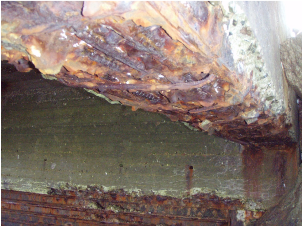
Figure 3 Corroded reinforcement bars with spalled concrete cover on a load carrying concrete beam in a quay deck.
